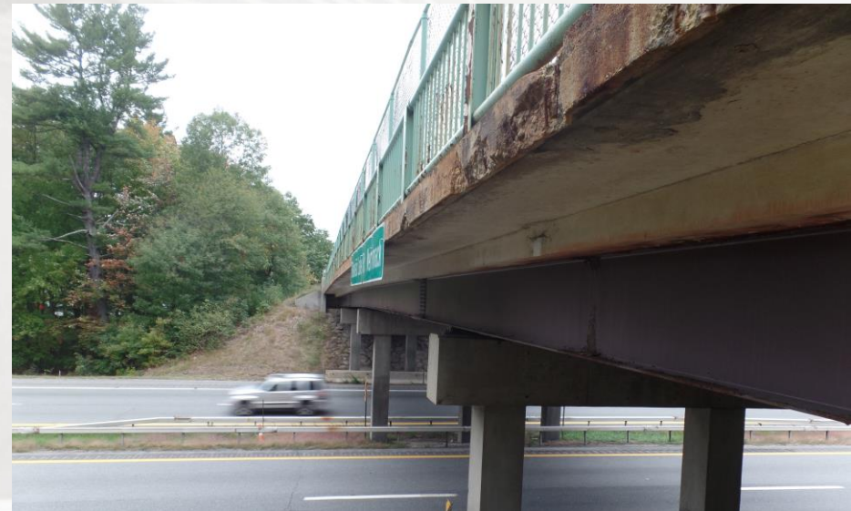
Existing 4-Span Bridge
